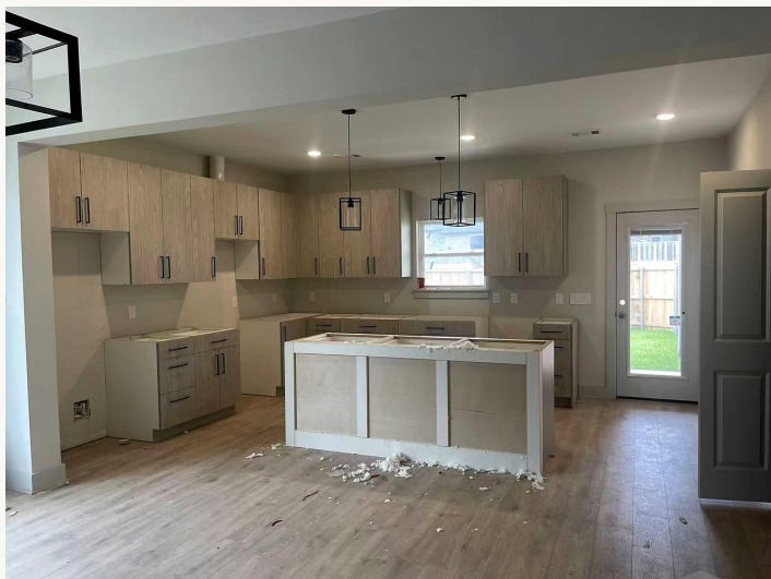
MID-INSTALL: CUSTOM WIDTHS THAT FIT THE ROOM
